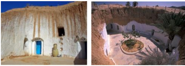
(b) Aerial view of a typical Matmata earth shelter dwelling.
