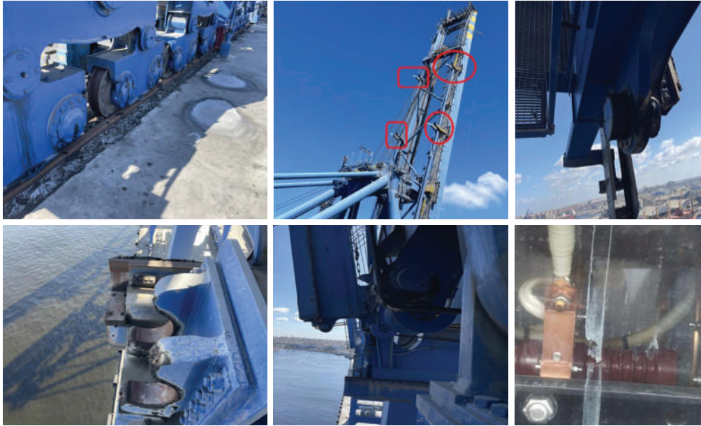
Figure 3: Level of damage in STS13 Source: Accident reports
