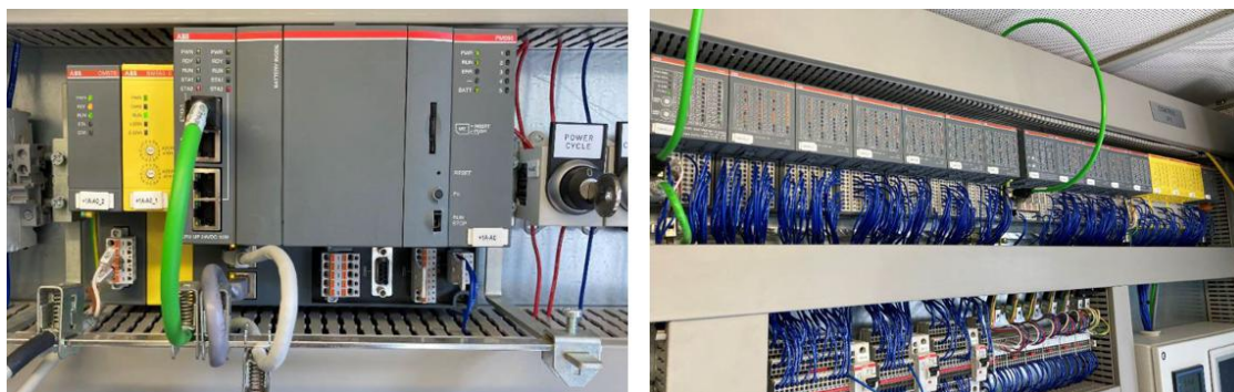
Figure 3. ERTG ABB PLC assembly on E-room including the remote I/O used for the pilot testing phase.
