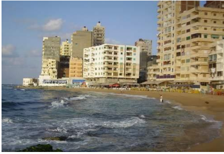
Fig .4. Presence of a lot of high illegal buildings on the waterfront
