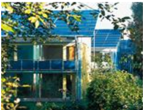
Fig .11. Each house has its own photovoltaic system to generate electricity
