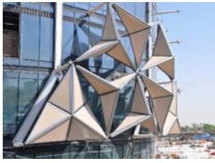
Fig .5. The folding and unfolding movement of the facade
