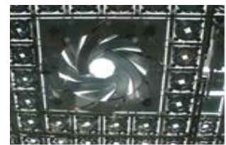
Fig .3. The dynamic circular shutter adopted from the traditional mashrabiya
