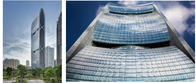
Fig .7. The dynamic façade of Pearl River Tower (China)
