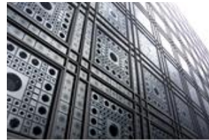
Fig .2. The façade of Arab Institute (Paris)
