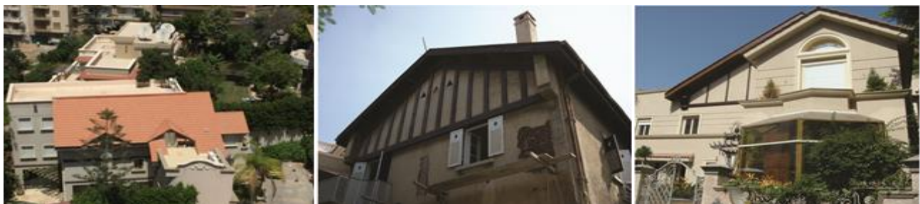
Fig .4. KafrAbdou villa (Source: author.) From Left: Arial Photo for villa in 2016. Middle: Villa before Rehabilitation. Right: Villa after Rehabilitation
