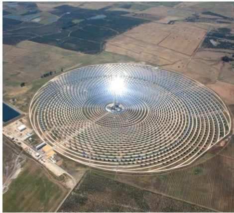
Solar Power Tower Technology, Gemasolar in Spain, 19.9 MW with 15 hours storage
