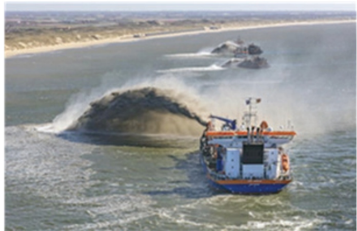
Figure 1: Developments in coastal engineering: change from hard designs (left) to softer more nature-based designs (right; beach nourishment, Netherlands). Hard structures with alien materials, like basalt rock, decrease natural properties of the coast (building in nature). Soft ones with local material, are more in line with coastal characteristics (building with nature).
