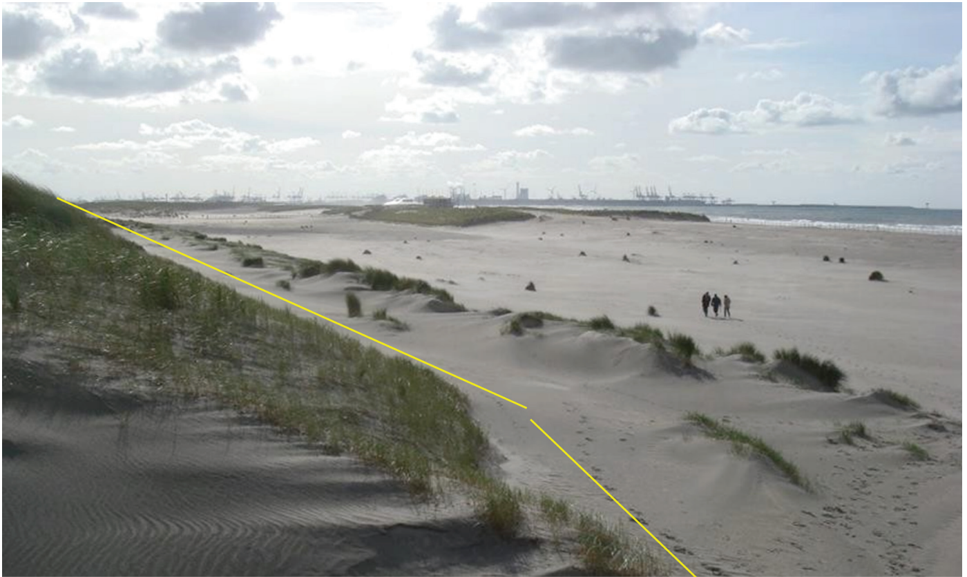
Figure 3: The new dune area, two years after construction (2011). Prospective dune marsh to develop in the lowest parts of the valley (middle). Prospective Grey dune to develop on the surrounding, more elevated sites. In the distance the new harbor extension of Rotterdam (Maasvlakte 2). Yellow line marks the border between existing dunes (left) and nourished dunes (right).
