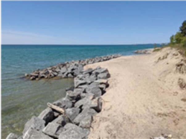
Figure 1: Developments in coastal engineering: change from hard designs (left) to softer more nature-based designs (right; beach nourishment, Netherlands). Hard structures with alien materials, like basalt rock, decrease natural properties of the coast (building in nature). Soft ones with local material, are more in line with coastal characteristics (building with nature).
