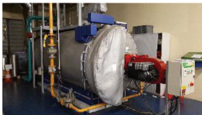
Fig. 3. Hot water boiler
