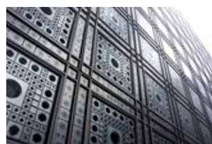
Fig .2. The façade of Arab Institute (Paris)
