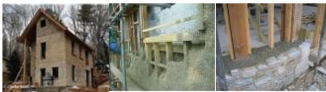
Fig.2. Shows that hempcrete can be cast manually around a timber frame using a shuttering system,
