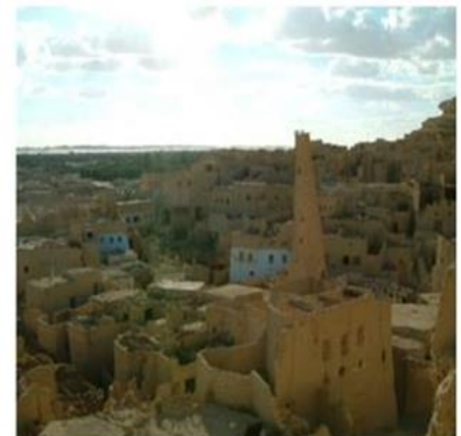
Fig.5.Architectural character of the Siwa Oasis [13].
